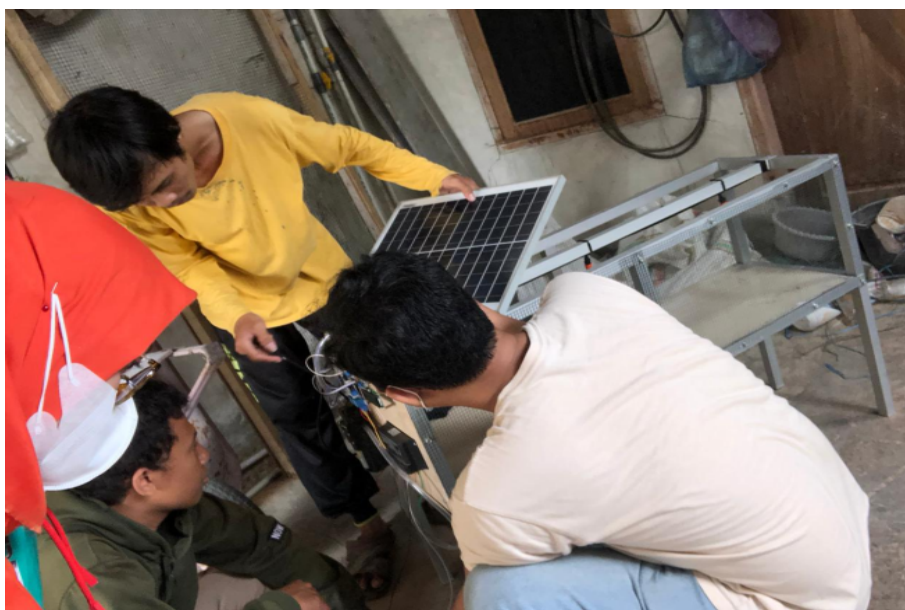
Fig. 3. Installation and assembly of tools
