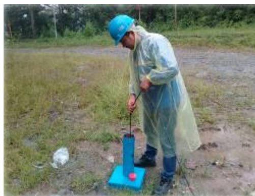
(c) Instalasi Piezometer
