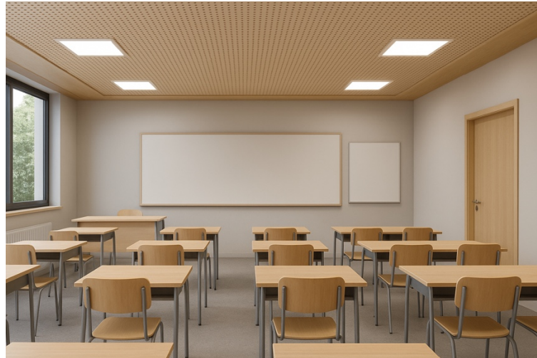
Figure 3. Interior classroom with perforated ceiling panels to improved acoustics Source: Siregar, 2025
